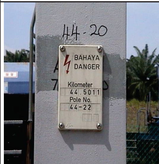
Figure 4: For KM below 0 or negative (-0); should be started with 10, i.e., 100379 (6 digits). For KM below 10; i.e., 1055 (4 digits). For KM above 10; i.e., 44500 (5 digits).
