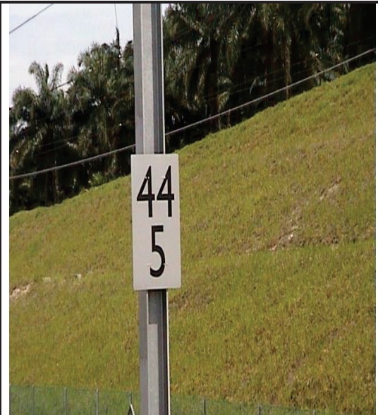
Figure 2: KM board stated the track position (KM) in sequence of XX.0, XX.2, XX.5, and XX.7.
