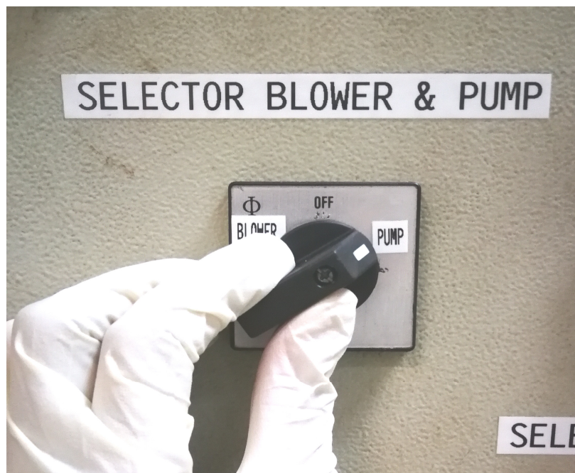
Figure 12.6: Switch the selector to ‘PUMP’
