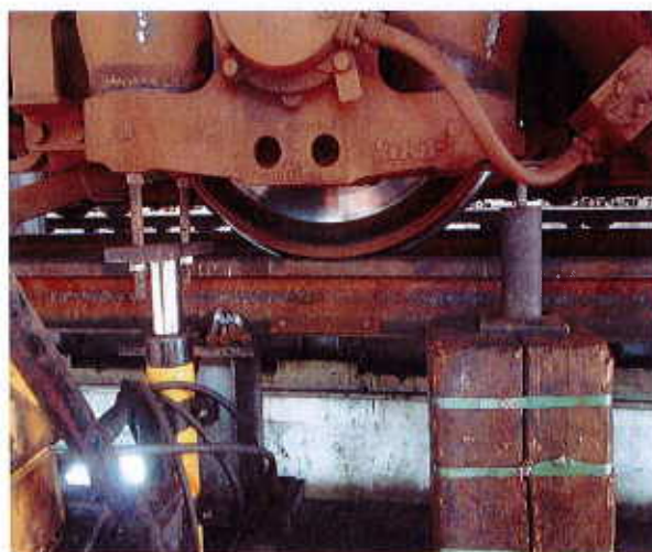
Figure 17 - Lift up the primary spring using hydraulic jack (2)
