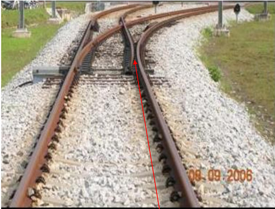
TURNOUT: SET TO RIGHT. Right Blade Open & Left Blade Close.
