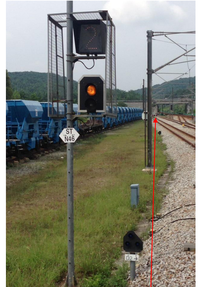
Entering Buffer End 1 Shunt Signal D2 Leaving Buffer End 1 Shunt Signal D1
