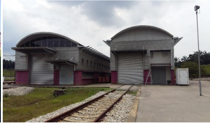
Track 8 Wheel Lathe & Spray Cabin
