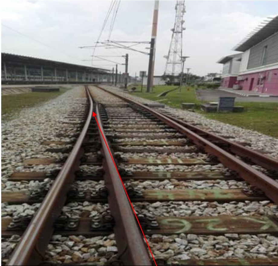
TURNOUT: SET TO RIGHT. Left Blade Open & Right Blade Close.
