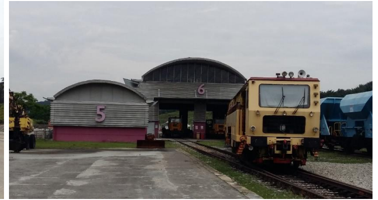
Track 8 Auxiliary Workshop
