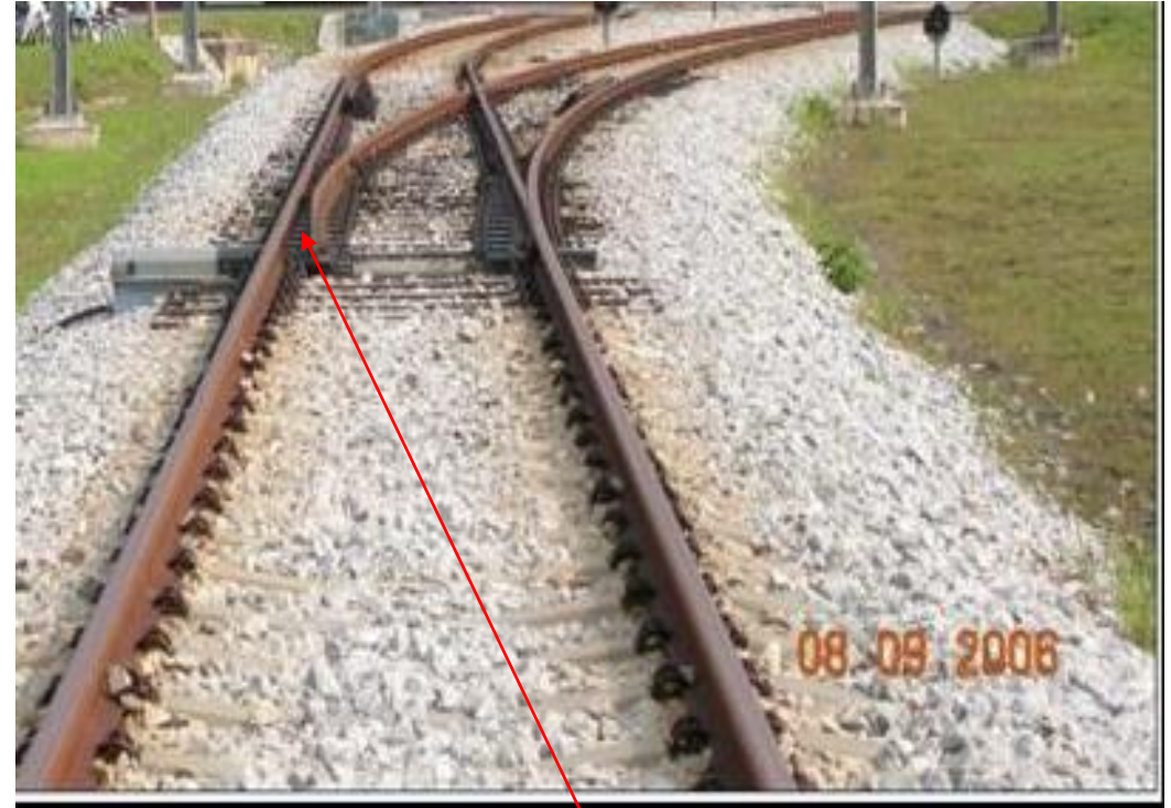
TURNOUT: SET TO LEFT. Left Blade Open & Right Blade Close.
